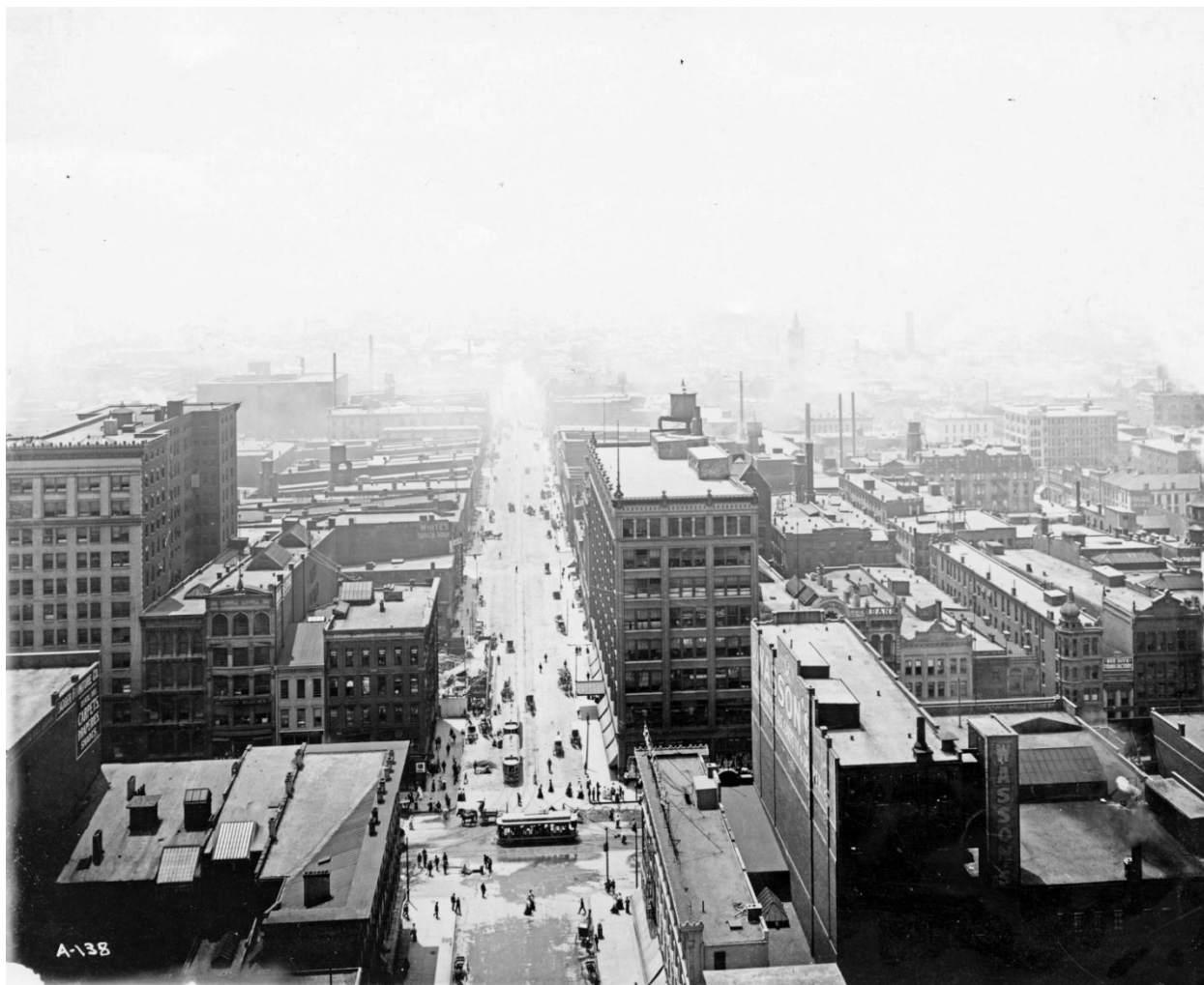
This image displays the penthouses, skylights, and water towers that littered warehouse rooftops in the IWD.
